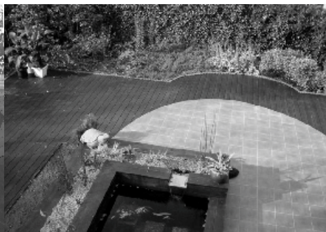
Two examples of decking installed finishing level with the surrounding ground. (No finishing border required.)
